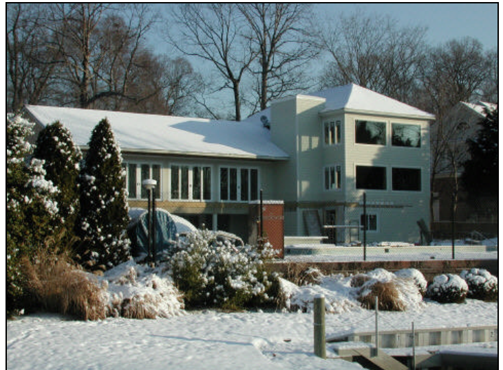
Snow now covers the MVYC Clubhouse, but the exterior is largely finished. Photo: George Holthaus
